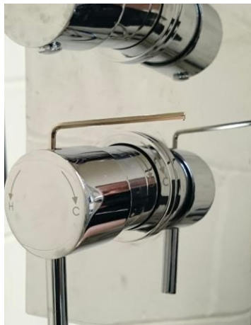
7. Again using the 2.5mm Allen Key, secure the Temperature Handle onto the Handle Bush.
