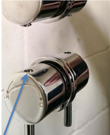
1. Remove the Temperature Handle Concealing Cap.
