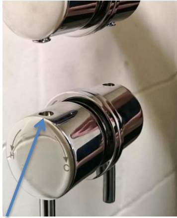
1. Remove the Temperature Handle Concealing Cap.
