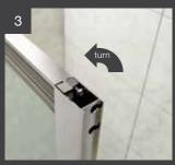
Secure screws into position using dedicated access holes.
