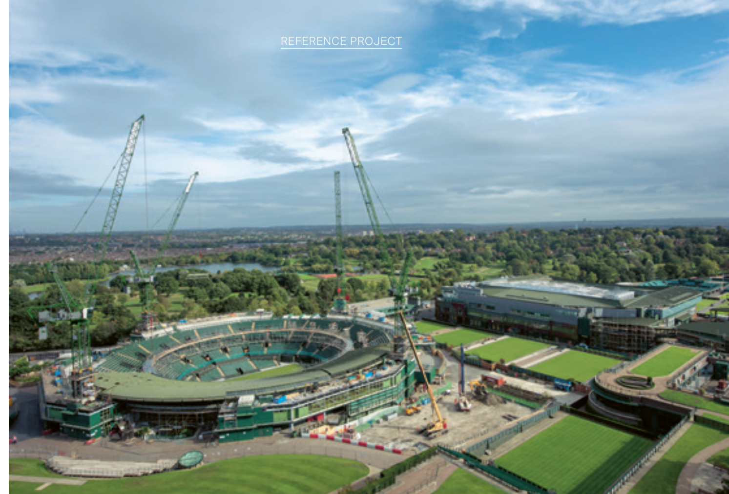
No. 1 Court at Wimbledon during the installation of the new roof elements.
