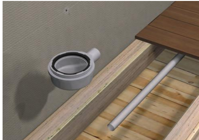
2. Install the waste ensuring adequate run off.
