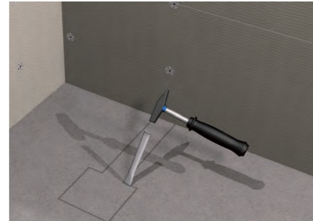
1. You will need to cut out the concrete floor to recess the waste and tray where appropriate.
