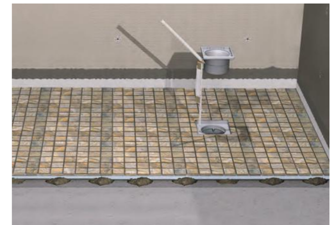
6. Your level access wet room is now ready to tile.
