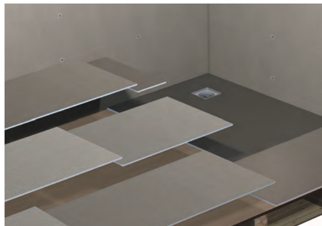
5. Fit shower tray and floor panels to entire floor area using board fixing adhesive and screws.
