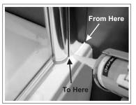
Seal down full height of wallpost to wall on INSIDE & OUTSIDE Seal junction of wallpost to bath on **OUTSIDE ONLY** as shown.
