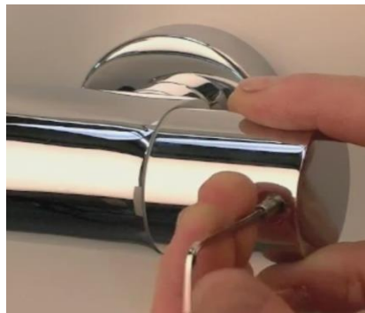
2. Using a 2.5mm Allen key, remove the Temperature Handle retaining grub screw.
