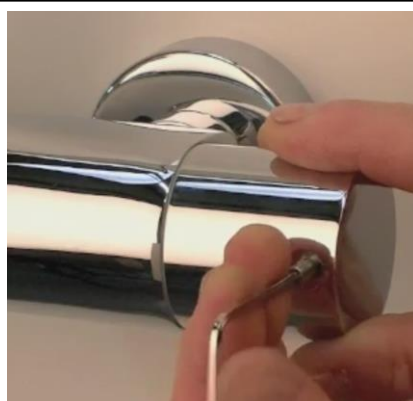
8. Again using the 2.5mm Allen key, re-attach the Temperature Handle.
