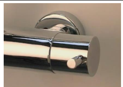
9. Re-fit the Temperature Handle Lever.
