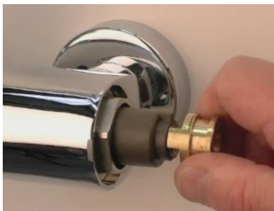
4. Relocate the Temperature Stop Lug back onto the Cartridge Spline by approx. 2-3mm in order to adjust the temperature.
