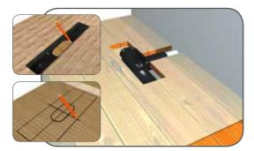
Measure the shower drain base position on the floor and mark this onto the relevant flooring.
